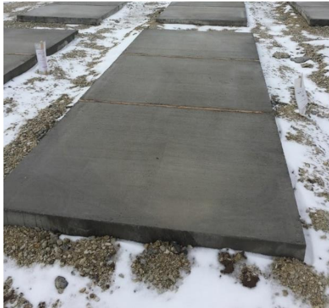
Figure 4-8: Center for Aging Infrastructure: Sidewalk Slab Exposure Site (January 2015)
