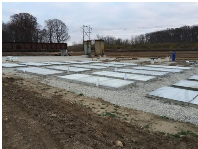
Figure 4-2: Center for Aging Infrastructure: Sidewalk Slab Exposure Site (November 2014)
