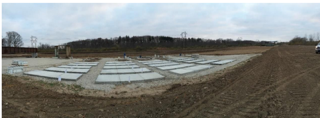
Figure 3-4: Panorama View of the Center for Aging Infrastructure: Slab Exposure Site
