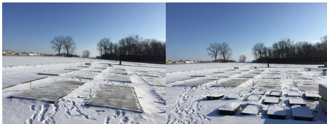
Figure 3-6: Pavement slabs undergoing freezing cycles at the CAI exposure site
