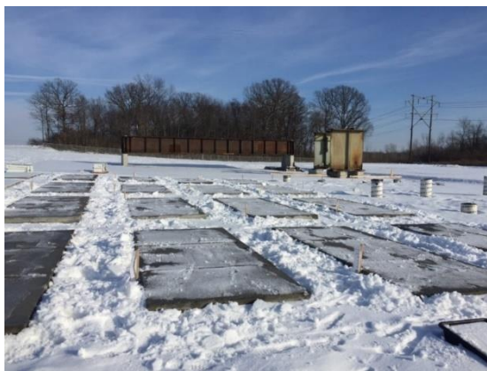
Figure 4-28: Center for Aging Infrastructure: Sidewalk Slab Exposure Site (February 2016)
