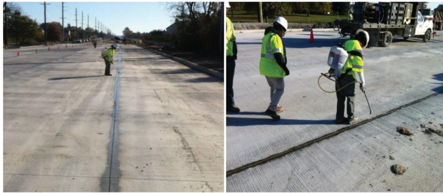
**Figure 2.17** Application of SME-PS to 126th street in Fishers, IN being performed by members of Berns Construction.
