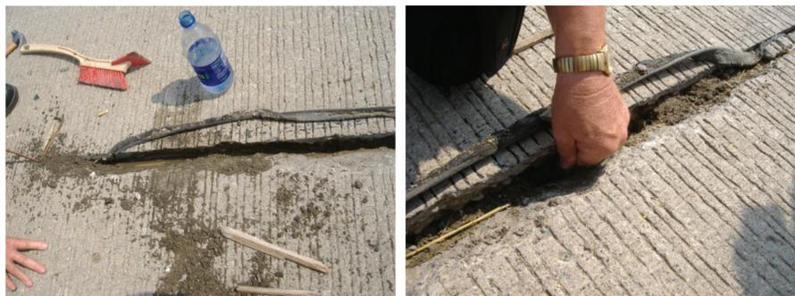
**Figure 1.2** Field observation showing damage in pavement joints containing water.
