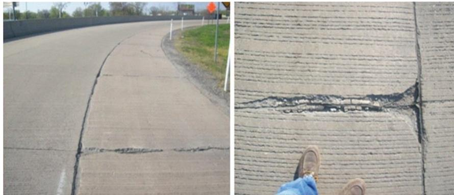
**Figure 1.1** Field observation showing damage in pavement joints.
