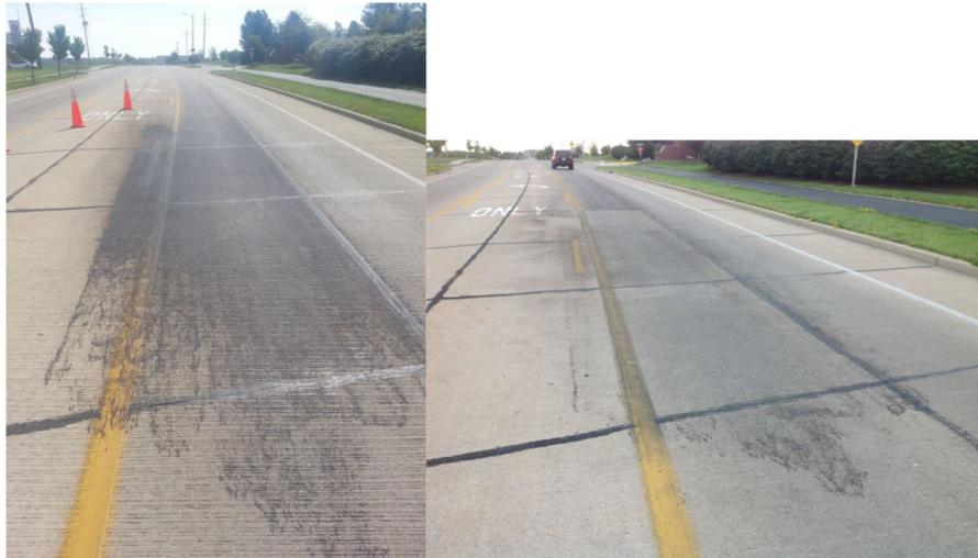
**Figure 2.11** Asphalt spill on Kalberer Road before and after removal using SME-PS.
